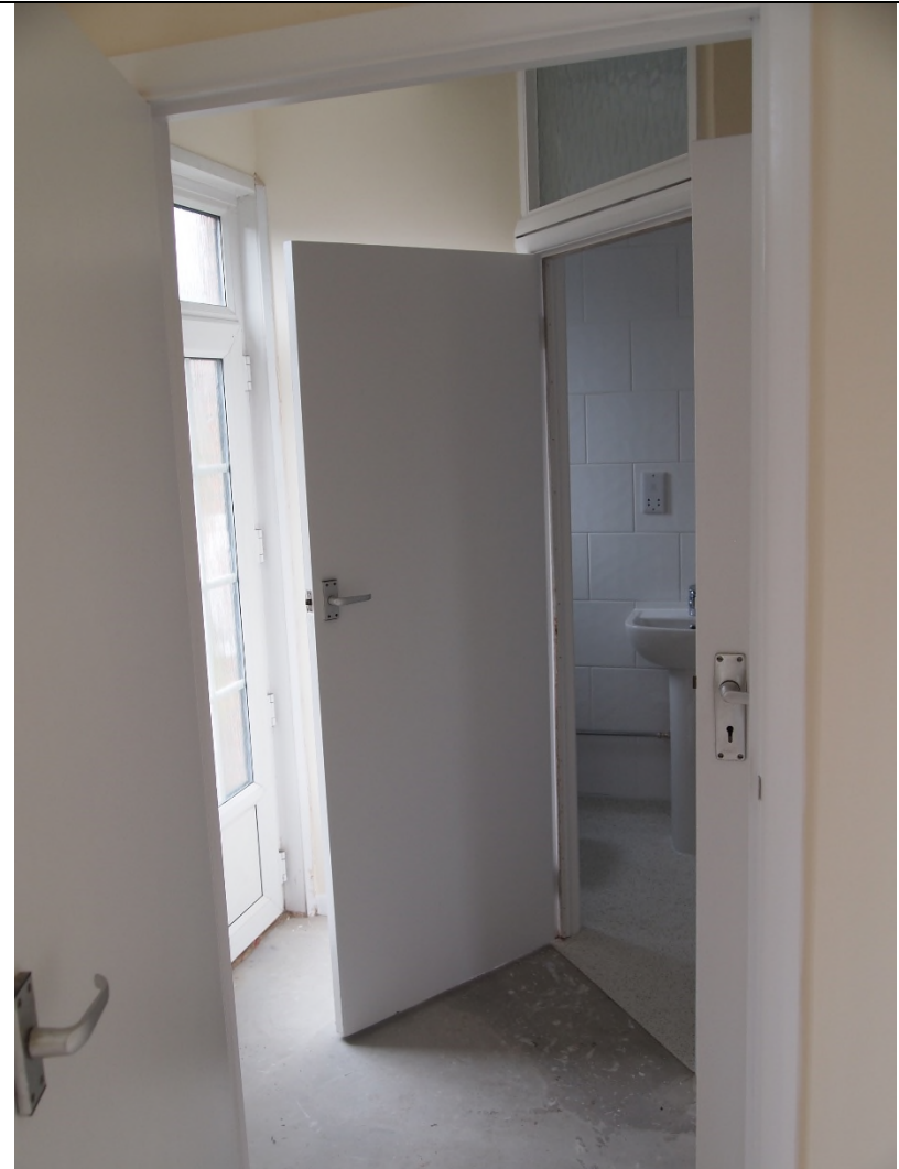
Rear hall showing the back door
