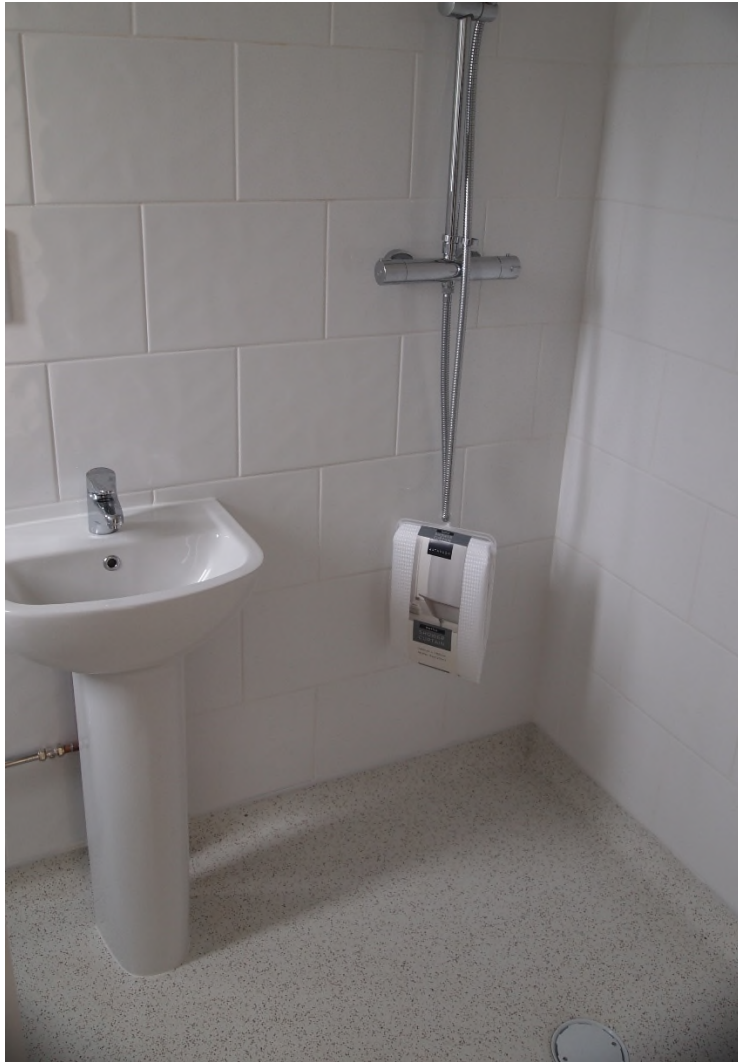
A walk in level access shower and toilet
